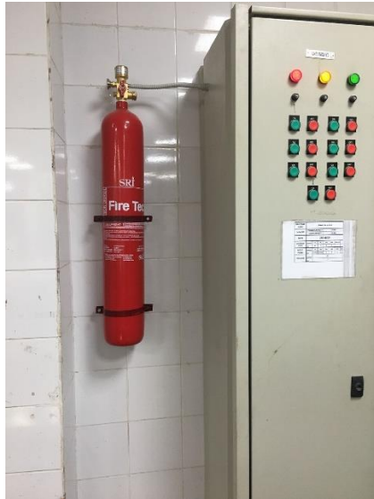
Upgrading our FM200 fire suppression system in both hotels
