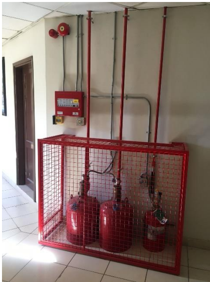
Upgrading our FM200 fire suppression system in both hotels
